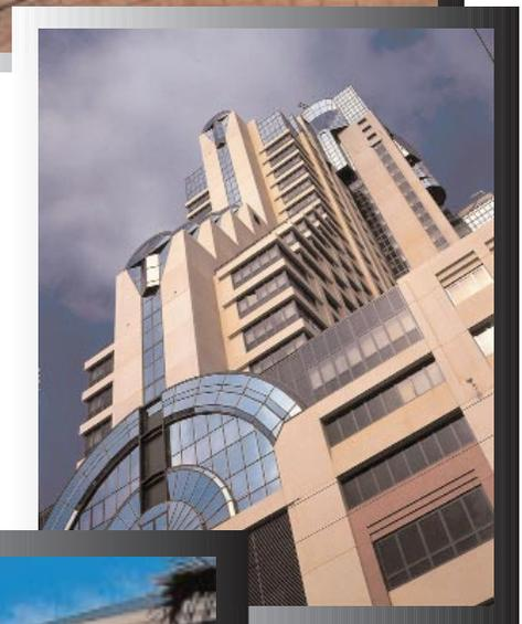
*Fig. 4. The San Francisco Marriott is built with precast panels made with white cement and a pink pigment. The upper floors are all glass fiber reinforced concrete. GFRC panels provide an attractive finish and are lightweight, strong, and durable. Architect: Zeidler Roberts Partnership, Toronto Canada. Photographer: Peter Leach, Denver, Pennsylvania.*
