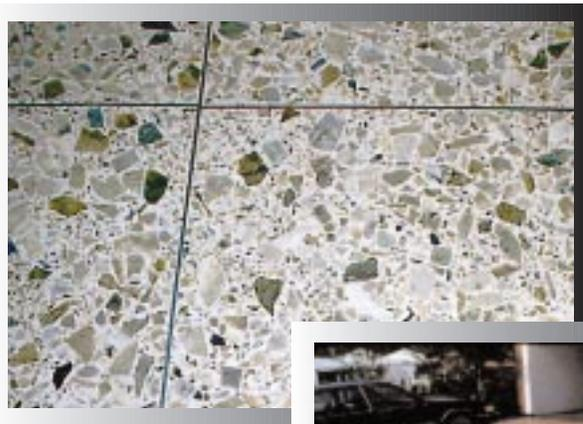
*Fig. 2. White cement complements any color. This polished terrazzo floor is made with white cement and green granite aggregate (#68923).*
